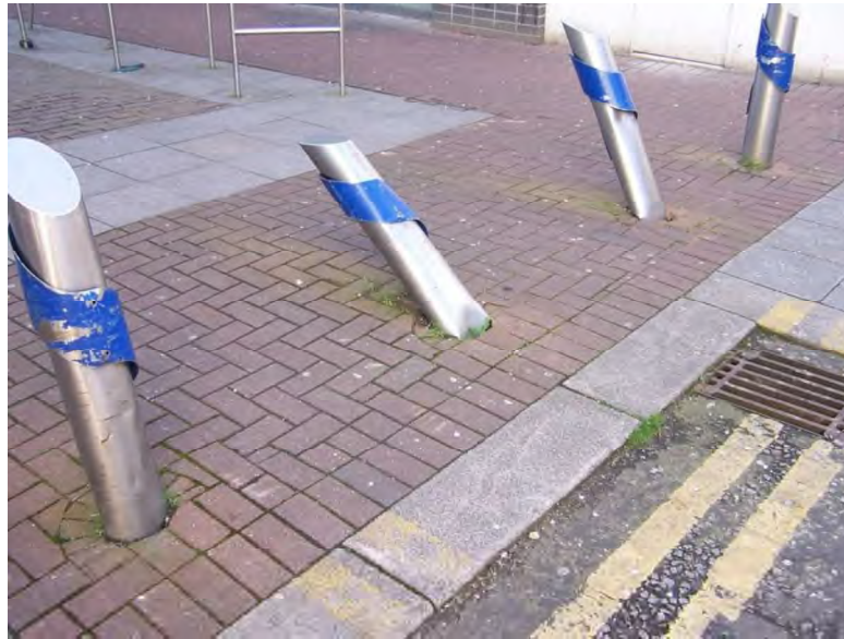
Figure 6: Route 5 impact point showing damaged bollards
